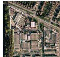
Power Towers's site in Leicester, UK.
